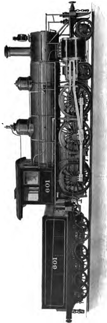
TEN-WHEEL PASSENGER LOCOMOTIVE SOUTH EASTERN RAILROAD OF RUSSIA.
