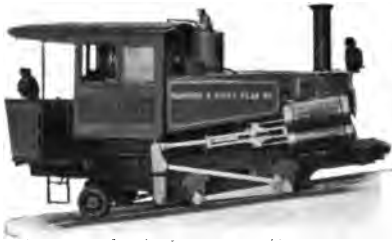
RACK LOCOMOTIVE, ABT SYSTEM.
