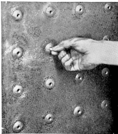
Installing Fireproof Porous Plugs in Tell-Tale Flexible Bolts
