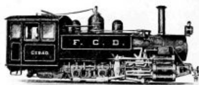
COMBINATION RACK AND ADHESION LOCOMOTIVE
