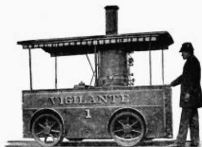
STEAM INSPECTION CAR
