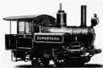
RACK LOCOMOTIVE, RIGGENBACH SYSTEM
