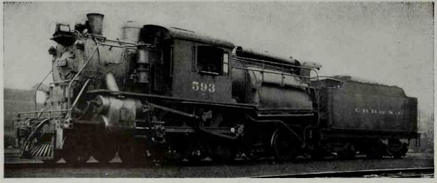
Central Railroad of New Jersey 4-4-2 (Atlantic) Type Locomotive, Class P-6, No. 593. Fast passenger locomotive built by the Brooks Works of the American Locomotive Co. in June 1902.
