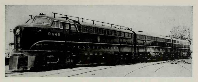
Pennsylvania No. 9448, Class FF-16, Three Unit, 4,800-hp. Freight Locomotive built by Fairbanks-Morse & Company in 1950.
