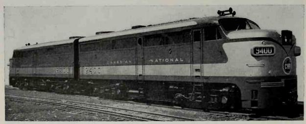
Canadian National Nos. 9400 & 9401, Class W-1-A; Two Unit 3,000-hp. Freight Locomotive built by Montreal Locomotive Works Ltd.—
