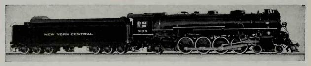
New York Central 4-8-2 (Mohawk) Type Locomotive for freight and passenger service, Class L-4a, Nos. 3100-3124 and Class L-4b, Road Nos. 3125-3149. Built by Lima Locomotive Works, Inc., in 1943.
