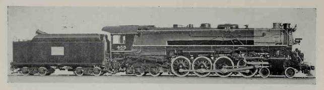
Central of Georgia 4-8-4 Type Locomotive, Closs K, for fast passenger and freight service, Nos. 451-458. Built by the Lima Locomotive Works, Inc. in 1943.
