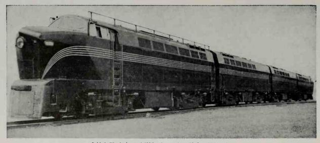
Baldwin-Westinghouse 6,400-hp. Locomotive with four RF-16 units.
