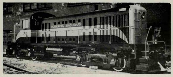
Roberval Saguenay No. 20, 1,500-hp. Road Switching Locomotive built by Montreal Locomotive Works Ltd.-Canadian General Electric Company Ltd. in December 1949.
