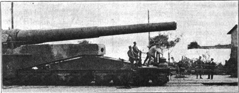
TRANSLATING MOUNT WITH HAND WINCH AND CABLE.
