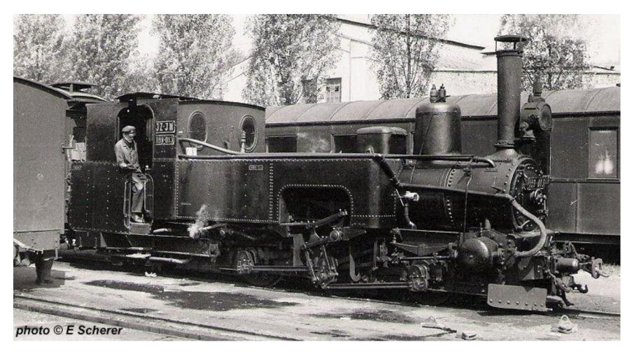
Klose fitted 0-6+2 tank 189-013 at Sarajevo, 3rd August 1965. There were 33 of this class of loco and they were introduced from 1885, the last one was withdrawn in August 1967.
